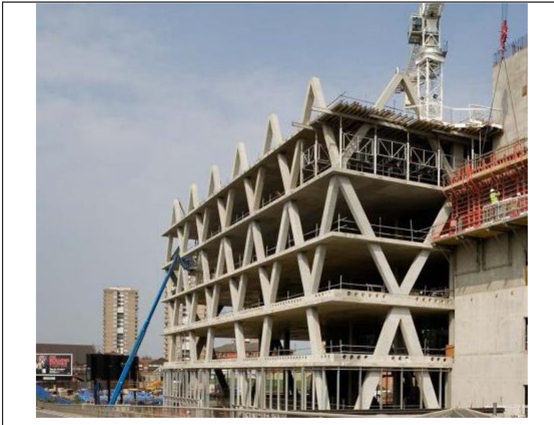
Figura 4.10: Edificio Yellow Building (concreto armado). Fuente: link https://www.ahmm.co.uk/projectDetails/8/The-Yellow-Building .
