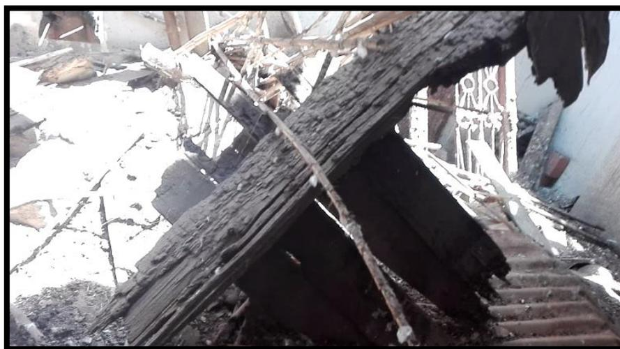
FIGURA 1.3 VIGAS DE MADERA CALCINADAS
